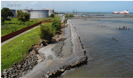
Ocean barrier created; Revetment wall constructed
