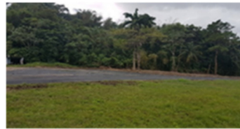
Site restoration and repaving
